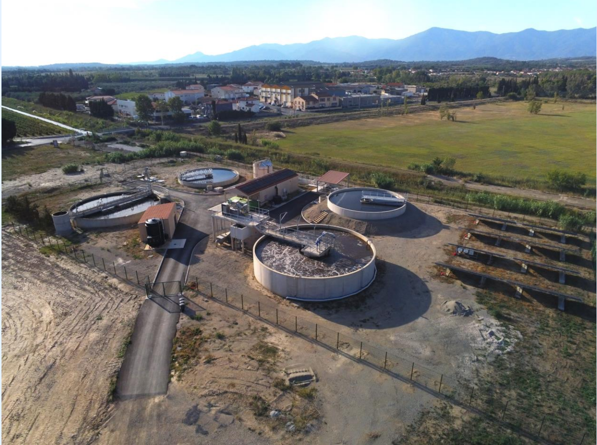
Extension station d'épuration - Bages
